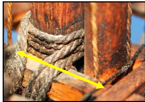
Figure 41: Absence of Bolsters
