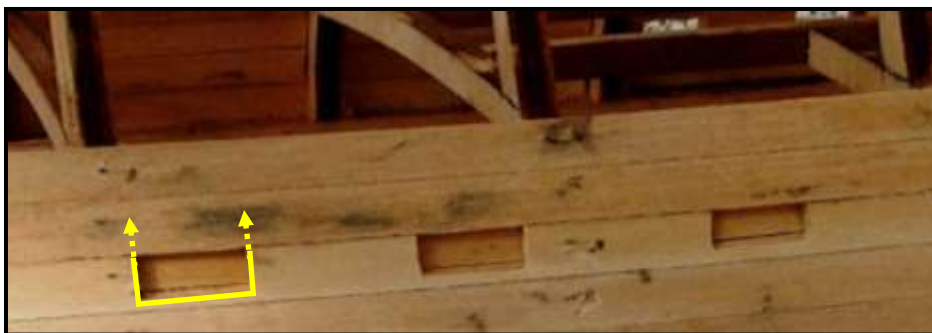
Figure 80: Beginning the Gunport Cut-Outs
