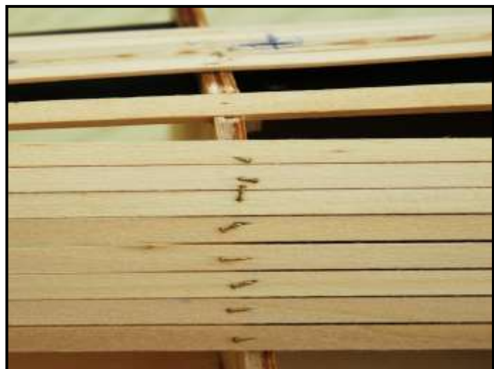
Figure 68: Drying Out Produces Gaps
