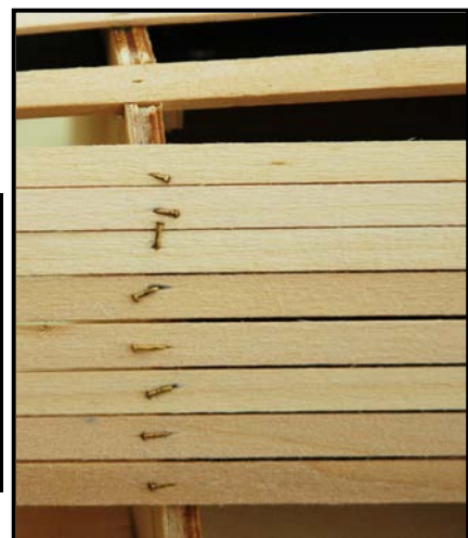
Figure 44: Drying of Wet Plank Results in Gaps
