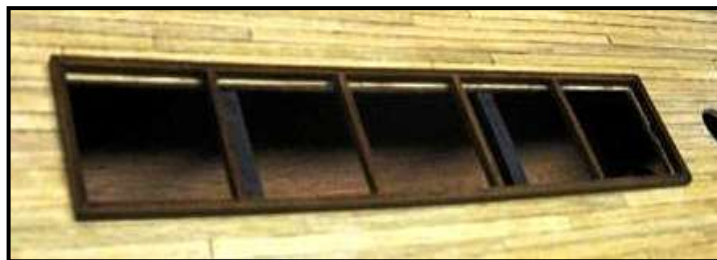
Figure 52: Outer Frame Constructed
